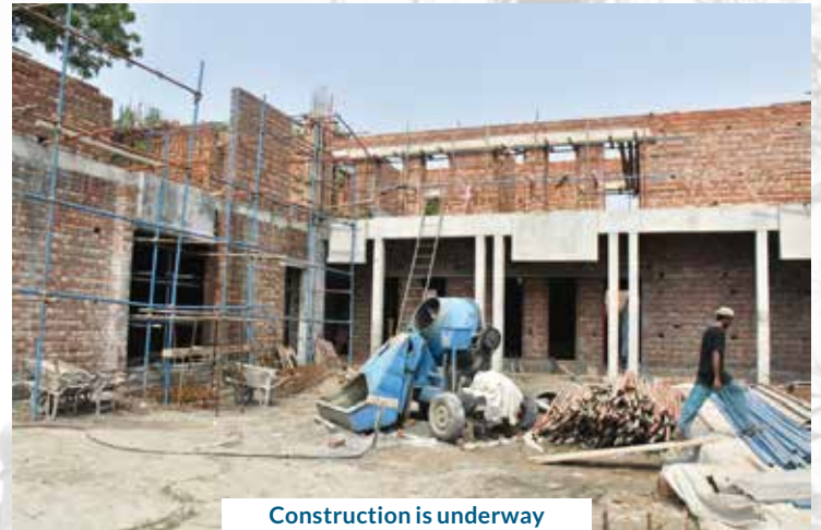
Construction is underway
